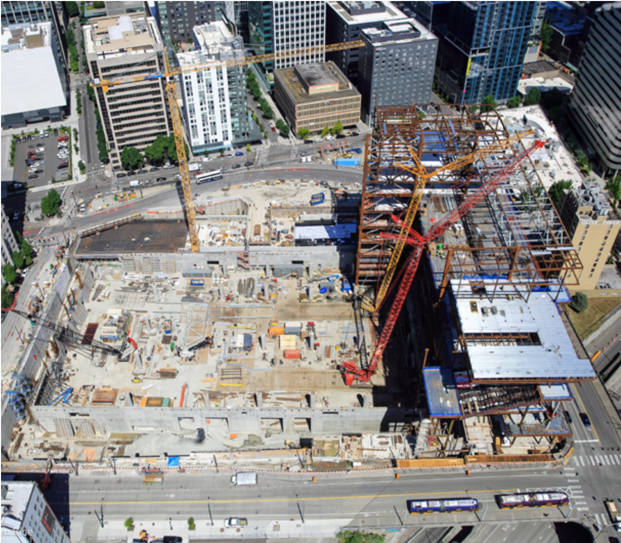
Summit construction photo illustrates the “billboarding” method.
